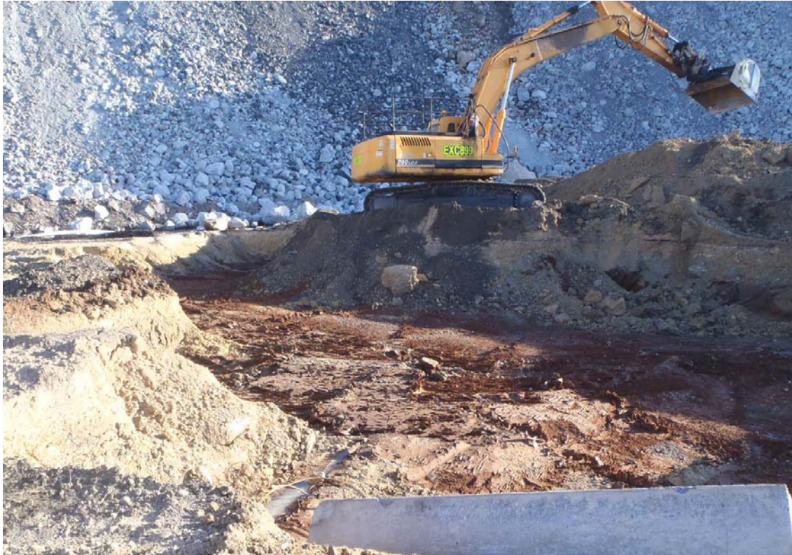
Figure 3.9 Excavator removing hydrocarbon contamination from the Former Workshop site
