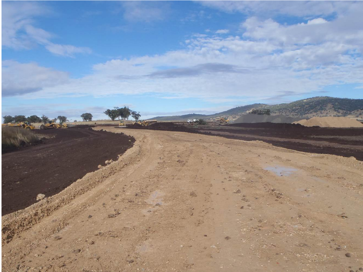
Figure 2.6 Equipment constructing the loop foundation layer of the Rail Loop Project
