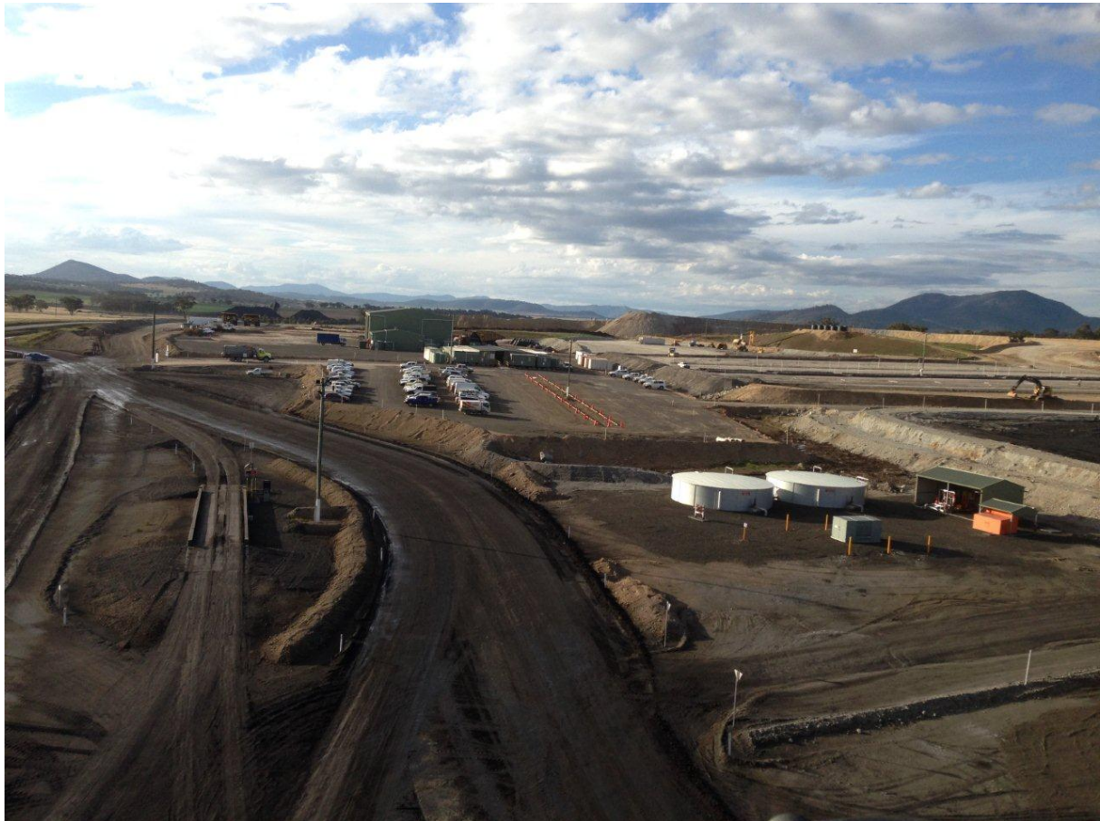
Completed Northern Mine Infrastructure Area (MIA) viewed from Truck Loading Bin
