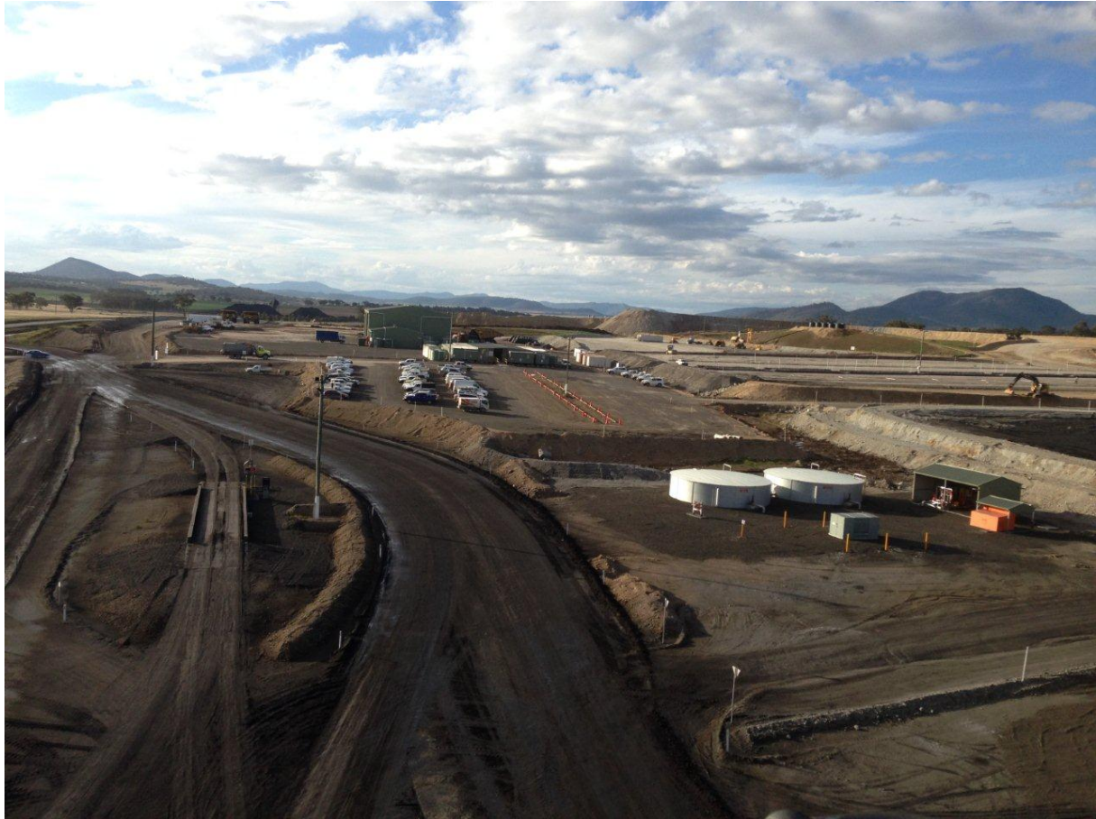
Figure 5.1 Completed Northern Mine Infrastructure Area (MIA) viewed from Truck Loading Bin
