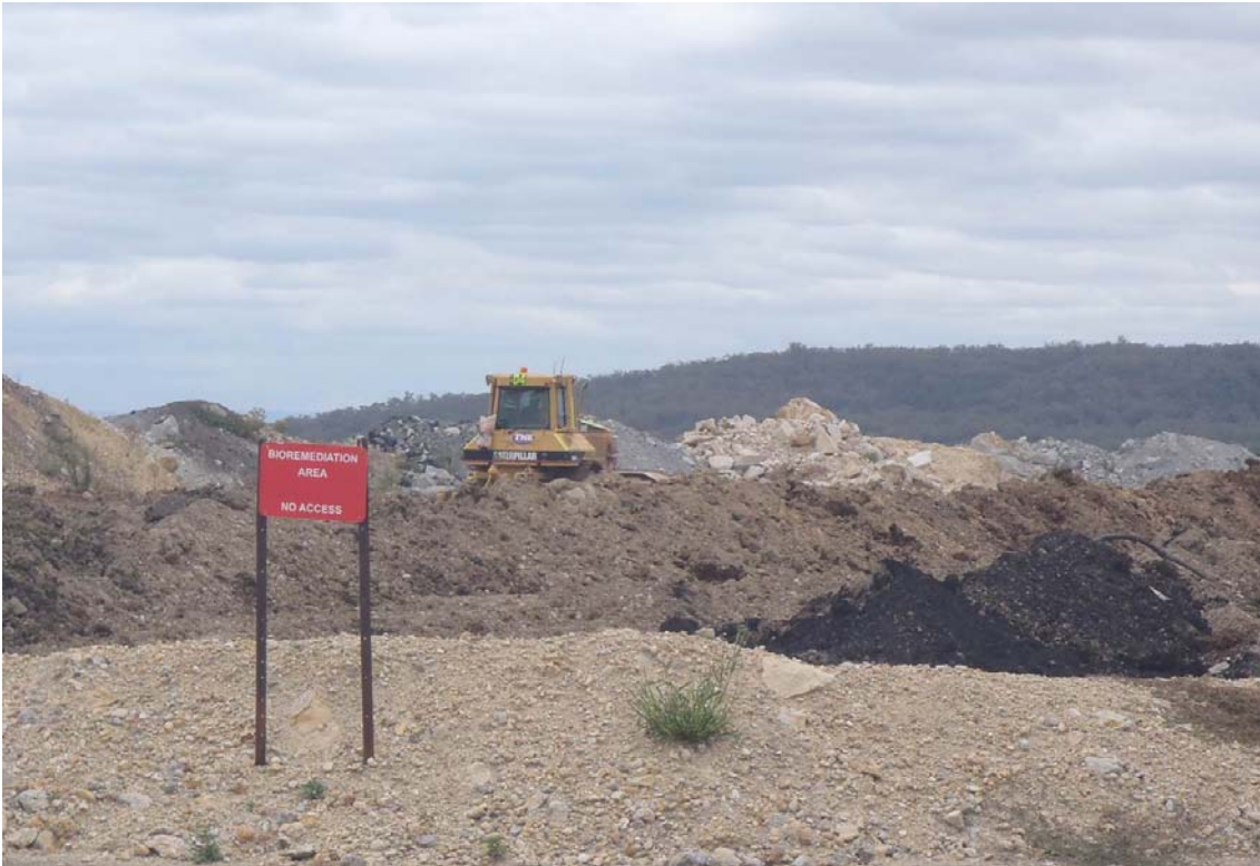
Figure 3.10 Dozer aerating and turnover contaminated soil in the Bioremediation Area
